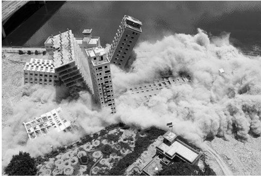
Figure 30: Blasting Demolition of Urban Village
