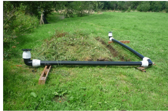
Fig. 4. Pipe rig just prior to burial.
