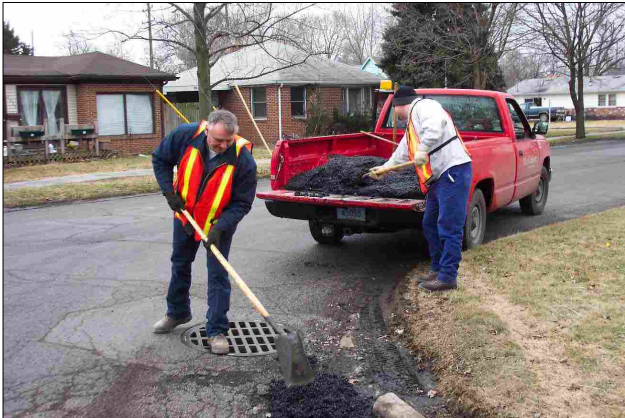
Figure 2.5 Example of cold mix asphalt patching [Layfayette]
