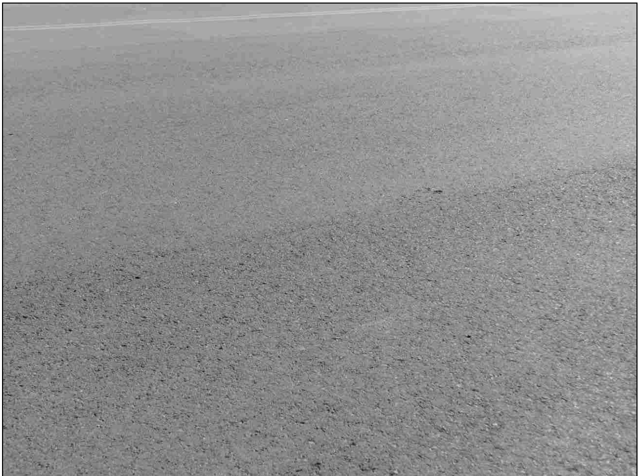
Figure 2.7 Example of HMA roadway surface
