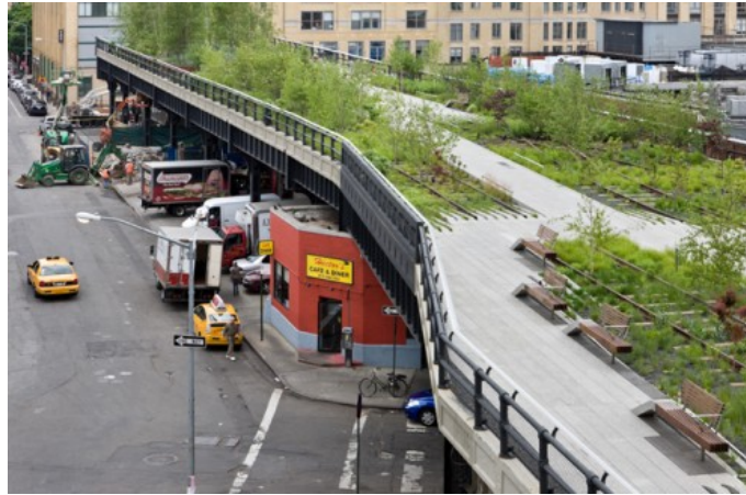
Figure 10: High Line Southern Terminus
