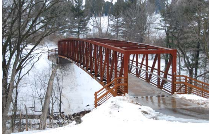
Figure 20: Box Truss Bridge
