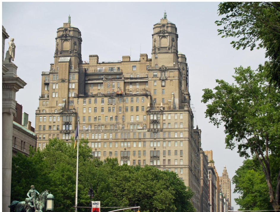
Figure 45. View of The Beresford Building
