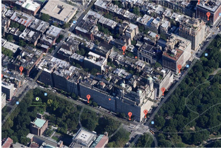
Figure 44. Aerial View of Amsterdam and 79 th Street
