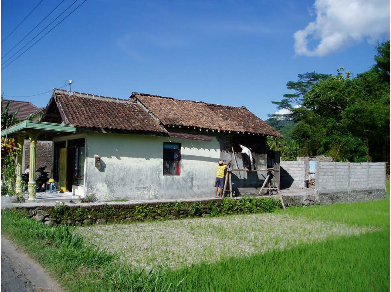
Figure 2: Self-Help Expansion of Home in Progress with Exterior Plaster Application
