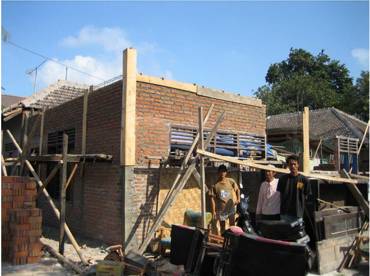
Figure 1: Typical Confined Masonry Frame Construction in Central Java
