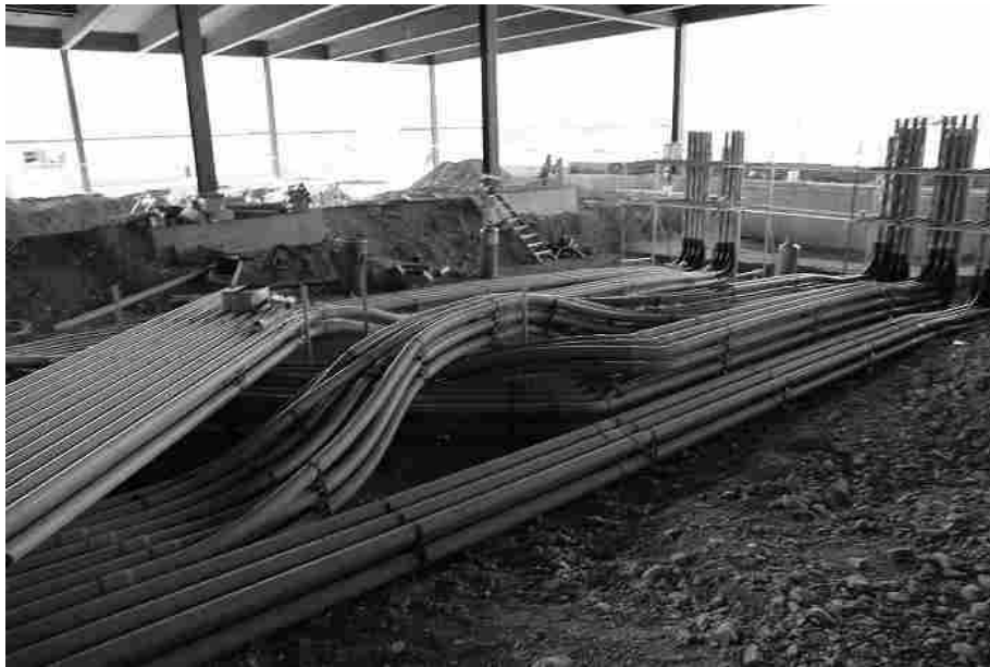
Figure 3.1.2: Underground PVC Conduit in Data Center Construction
