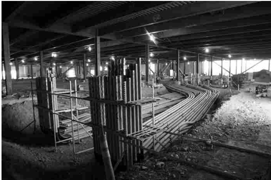
Figure 3.1.1: Underground Conduit in Data Center Construction
