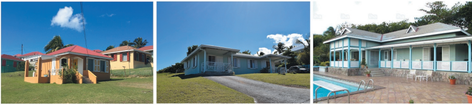
Figure 2. Housing in Montserrat. From left, a concrete block house built at Lookout, a Force 10 prefabricated house at Lookout and an upscale villa at Old Towne (Sources: Left and center, Ross Eisenberg, licensed under CC BY 4.0; Right, “Luxury villa” by Member #56594, licensed under CC BY 4.0).
