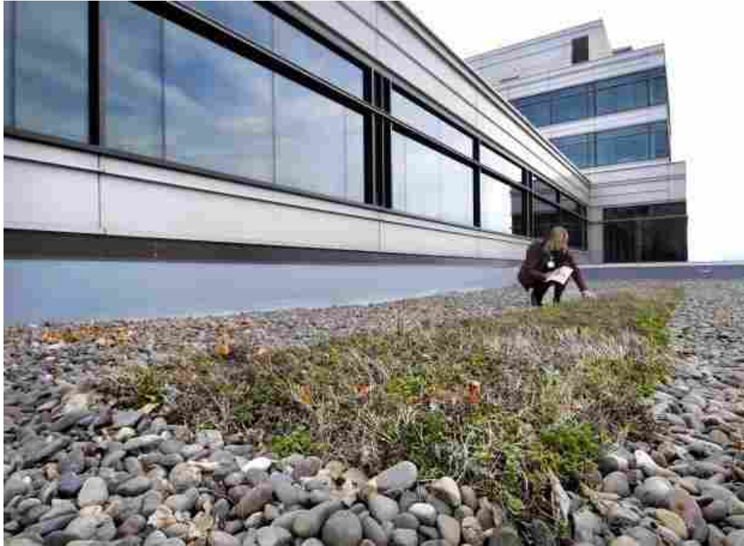
Figure 3: A demonstration extensive green roof sedum strip atop St. Patrick Hospital, Missoula. Photo via www.missoulian.com .
