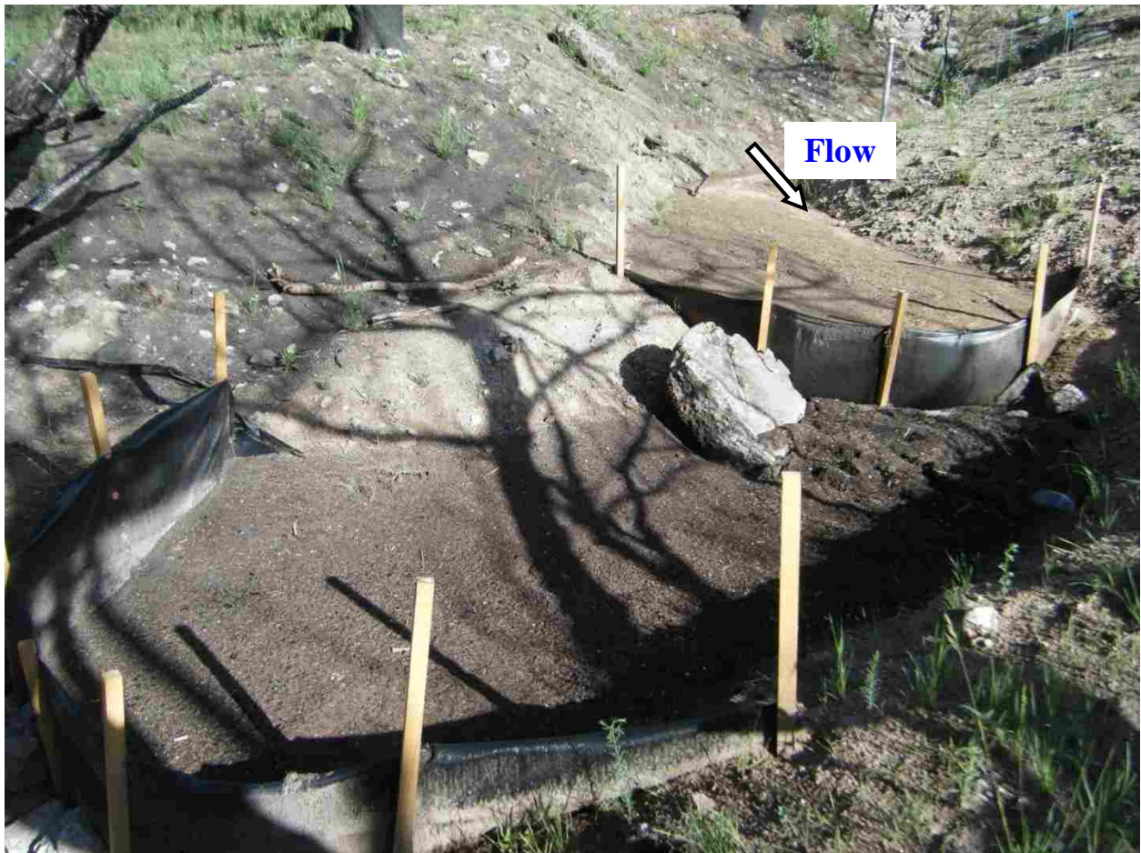
Figure 13. Total sediment yield captured by sediment retention structures in catchment I.5 from an event on 8 July 2011. Lower sediment yields in Middle Canyon allowed total annual sediment yields to be captured during the 2011 monitored period.
