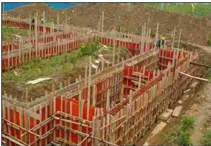
Figure 4.7: Concrete Form Construction in China
