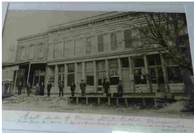
Figures 2.6, 2.7, 2.8: Bethel Colony businesses, photographs of prints in Bethel, Missouri taken by the author
