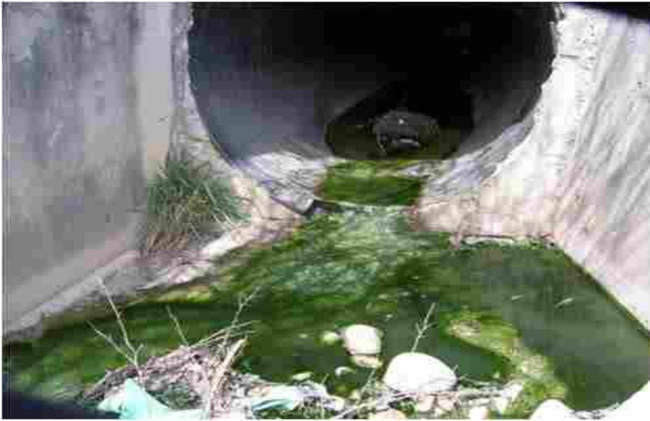
Figure 1.5: An example of contaminated small drainage by effluents near one garrison under command of 3rd division at Kangwon province (CWinews, 2009).
