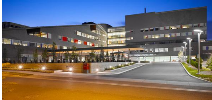
Figure 11. Bloorview Hospital, Canada, Exterior, http://www.metropolismag.com/story/20080220/health-and-happiness
