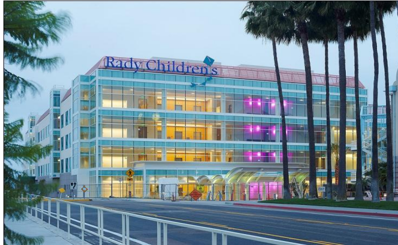
Figure 18. Rady Children's Hospital, Exterior, http://www.rchsd.org/
