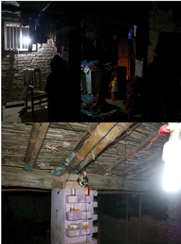
Figure 3. A lightbulb installed on the window to light multiple spaces (top). A bulb with plugs for charging mobile phones and spaces created for them (bottom).
