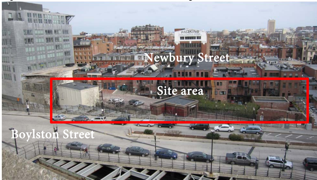
Figure 18: View of the site from the south, looking north
