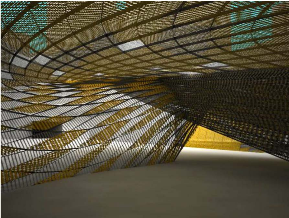
Figure 13: Structure and grated decking serves as a walking surface on the exterior above while providing shading and screening below.
