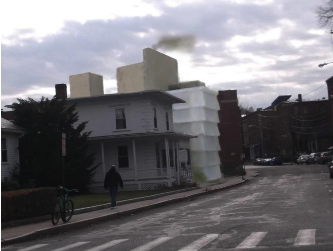
60 Masonic Street, Northampton MA
