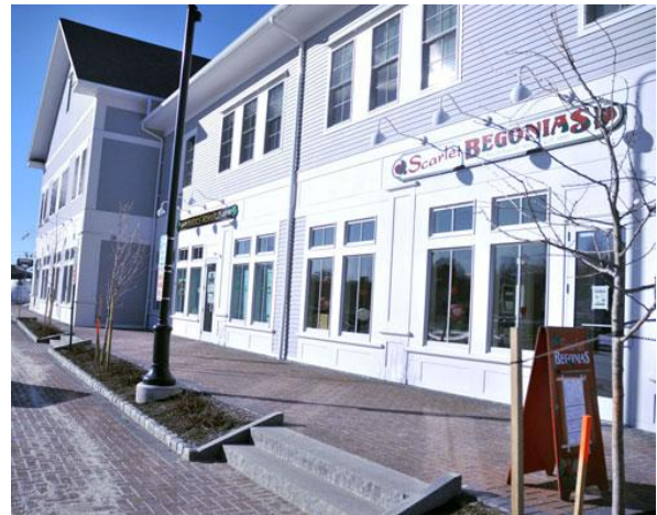
Figure 6: Maine Street Station, mixed use building, City of Brunswick, ME
