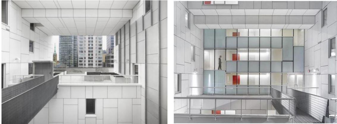
Figure 7 - Interior Views of Central Passive Ventilation Shaft
