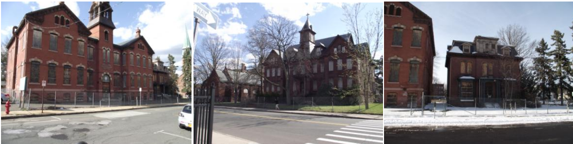
Figure 30 - Existing Catholic School Buildings on Site
