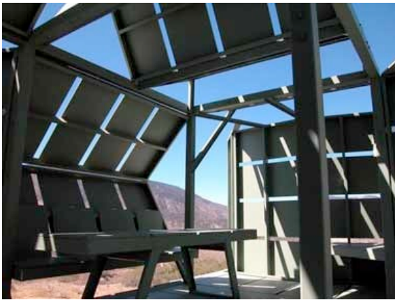
Figure 14: M-House Semi-Enclosed Exterior Space
