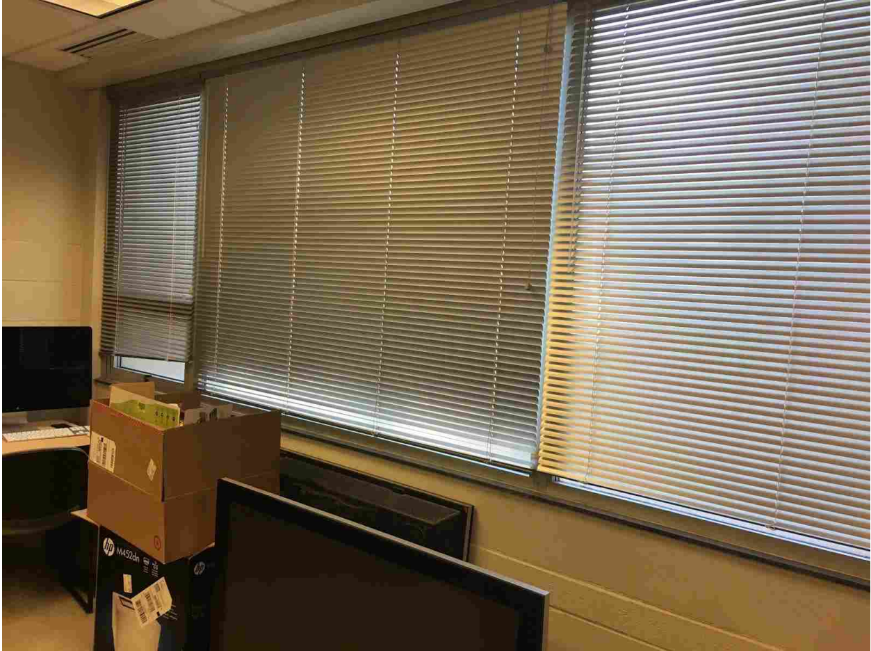
Figure 4.5. Blinds-covered windows filtering out direct sunlight. Photo by author.
