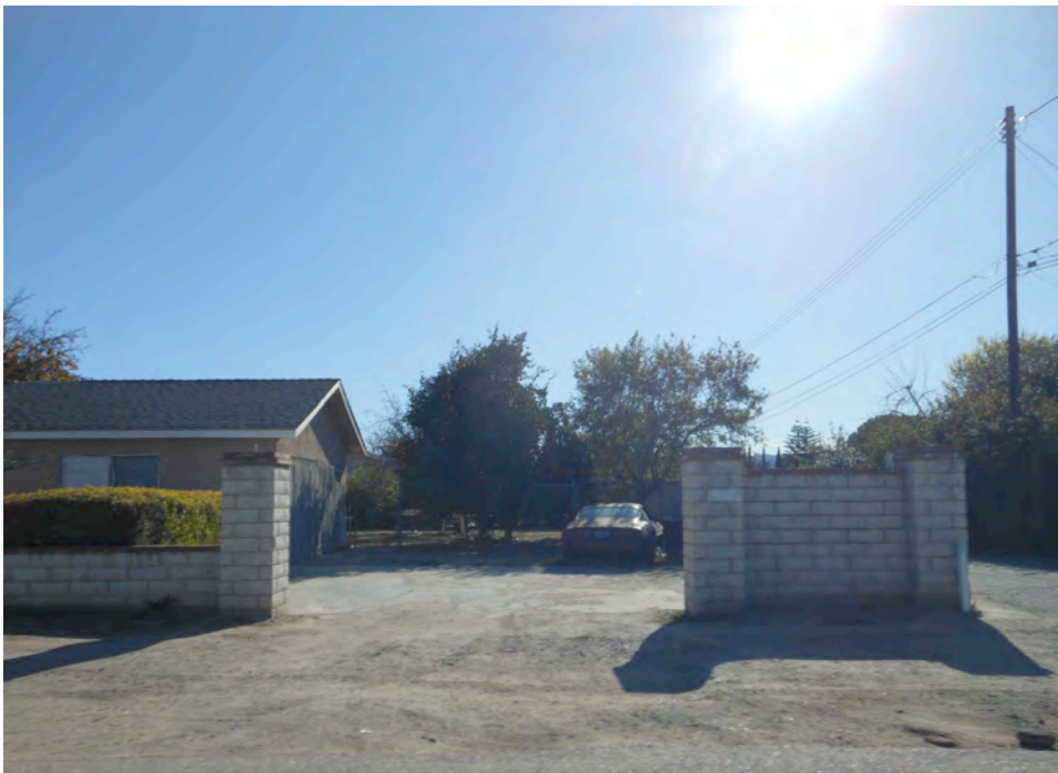
Figure 42 – Concrete Block Wall by Author.
