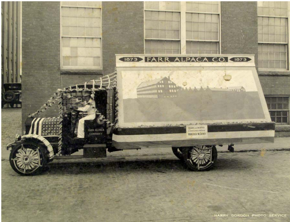
Figure 13. Behind the truck, the original and still intact glazing system (courtesy Holyoke History Archive)
