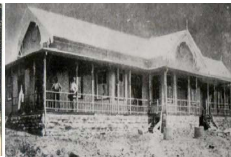
Fig. 2 "The Big House," in Pretoria, during the course of erection 1909 2
