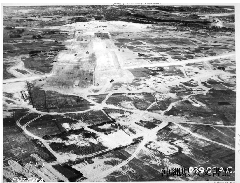
Figure 2. Futenma Air Base under construction. The image was taken on 30 June 1945. Source: Okinawa prefectural archives.
