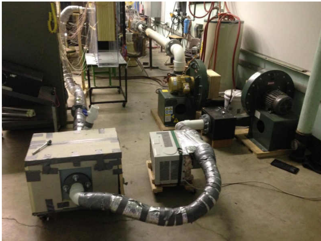
Figure 25. Entire coolant supply system.
