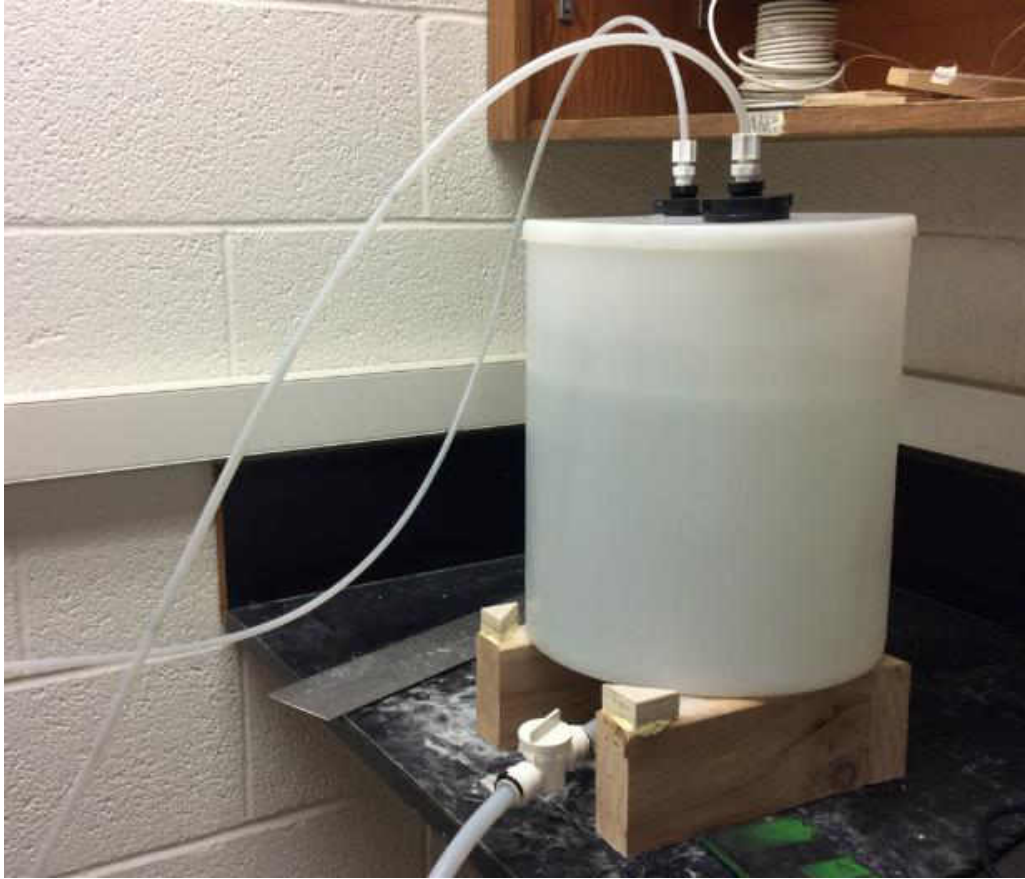
Figure 30: The DI water storage tank
