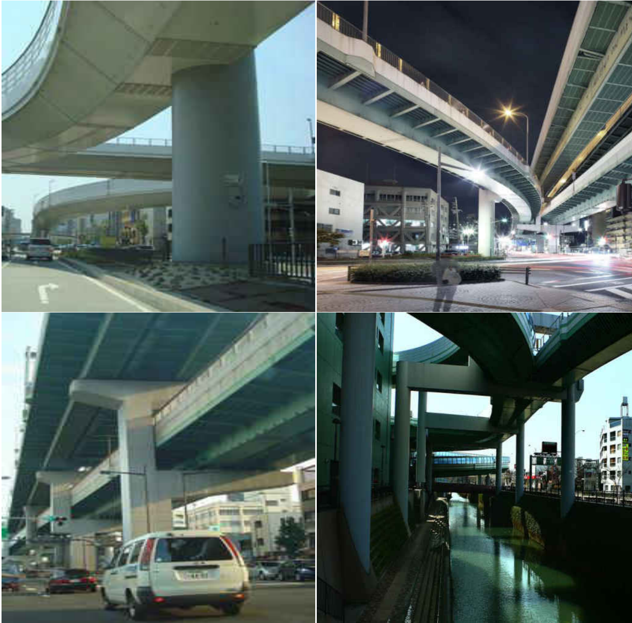
Fig. 1.1. In-service Steel Bridge Piers (Courtesy of Google).
