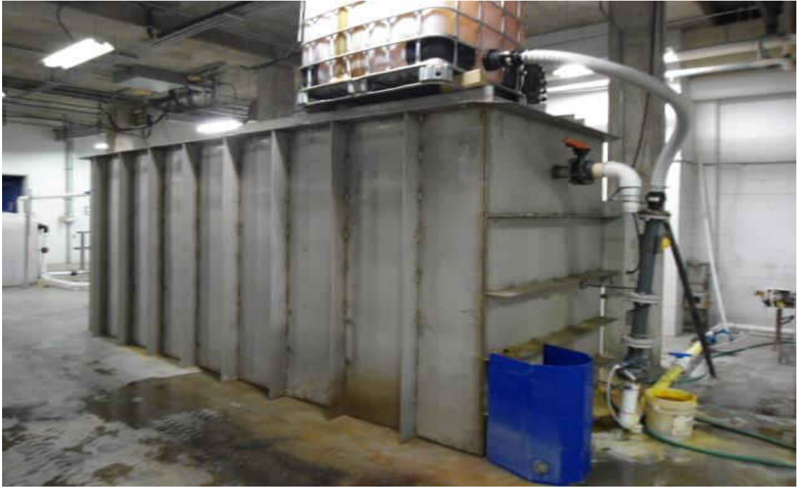
Figure 4.5.1.1. Pretreatment unit: MRI pretreatment, Raw water, acid and PACl feed point, and static mixer.
