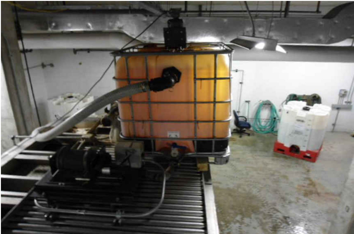
Figure 4.5.1.2. Mixer for coagulation.
