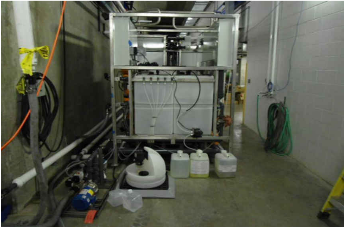
Figure 4.5.3.2. Rear view of the ultrafiltration unit from Evoqua.
