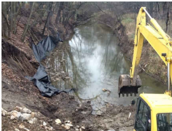
Installing rock along river toe
