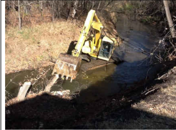
Removing fallen trees from the river
