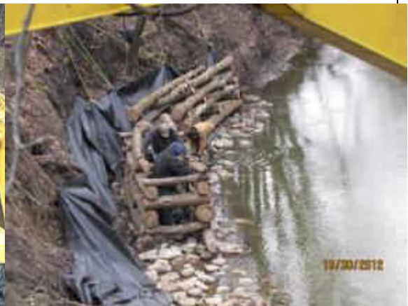
Installing cribwall on rocks
