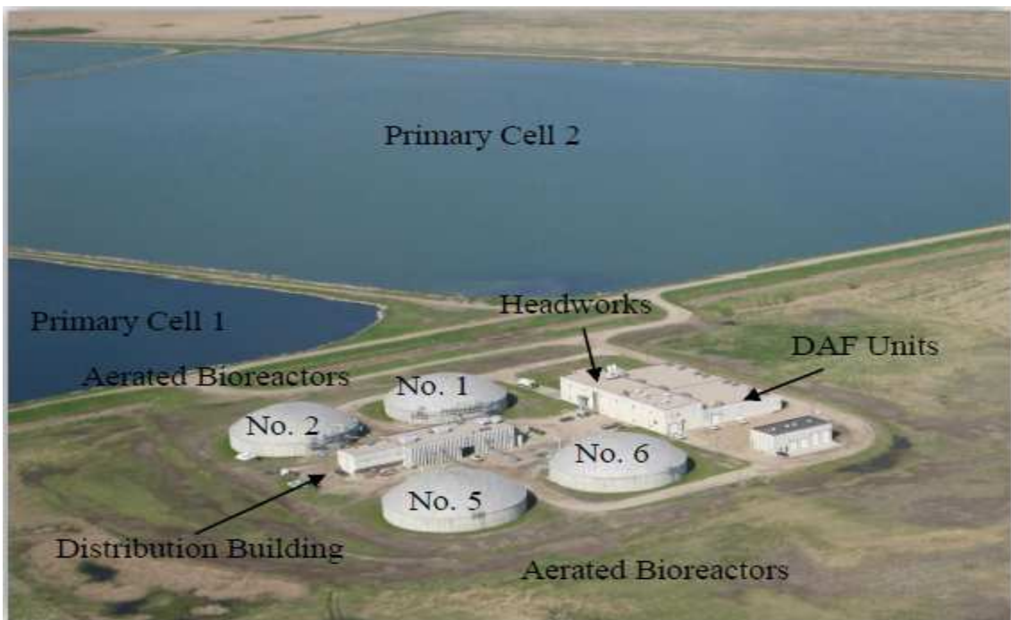
Figure 2-1: Aerial Photo of GFWWTP
