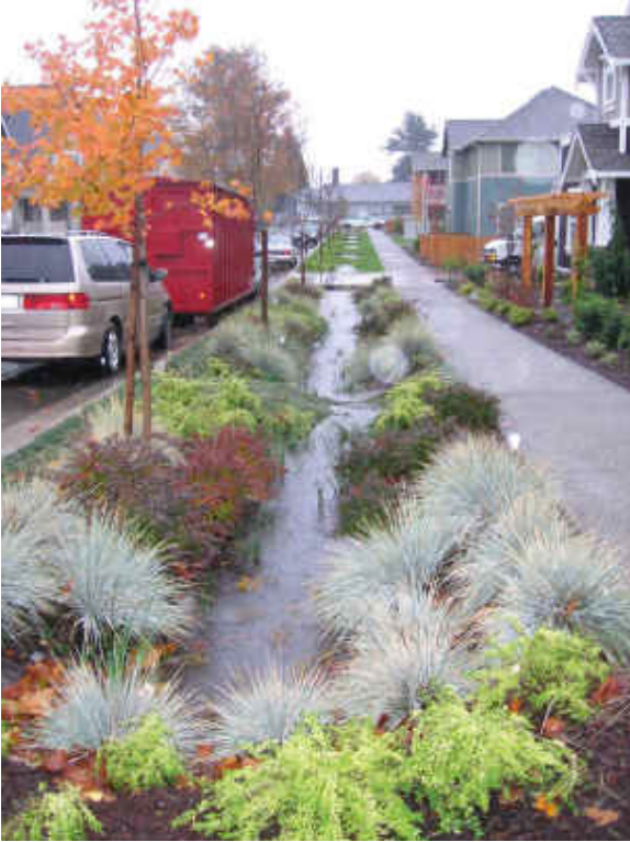
Figure 4: Bioswale (Source of image: Michigan Water Council)
