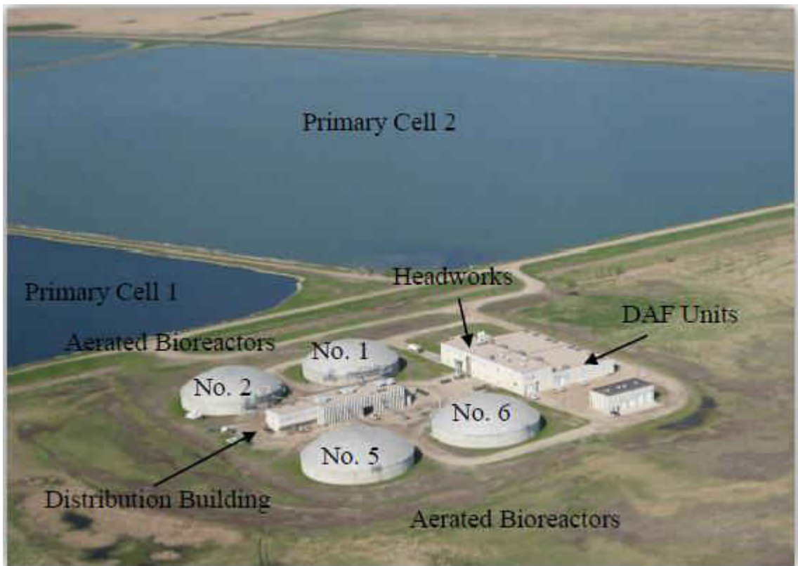
Figure 2.1: Aerial Photo of GFWWTP Source: (Kistner, Brian T, 2011)
