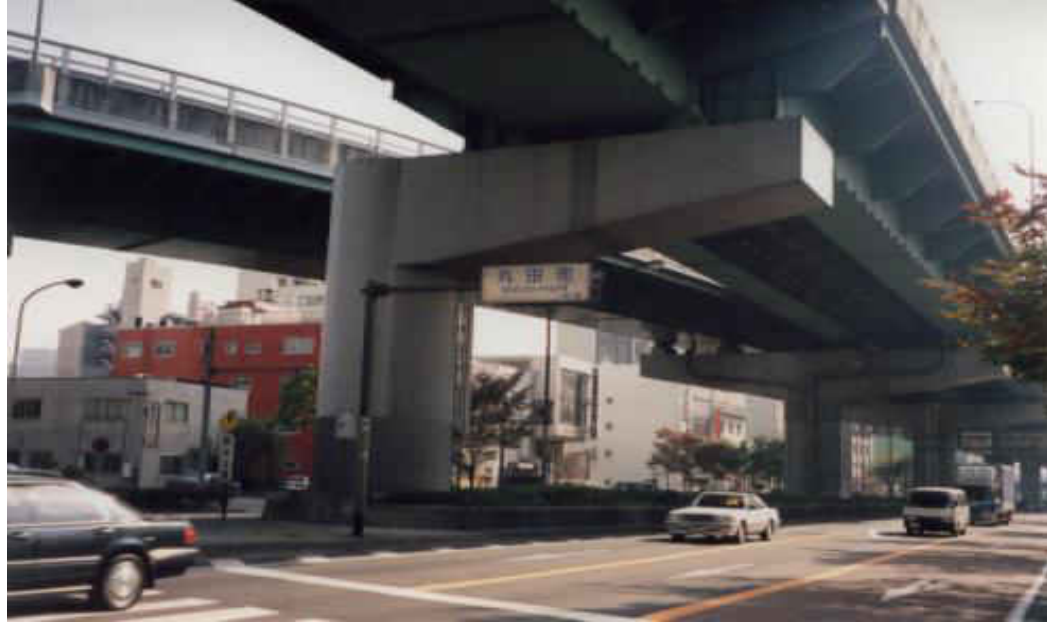
Figure 1. Thin-Walled Steel tubular Columns Supporting Elevated Highway Bridge in Nagoya, Japan.
