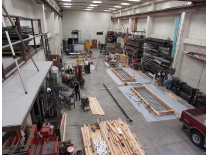
Figure 3-4: Footing Reinforcement Cages and Forms
