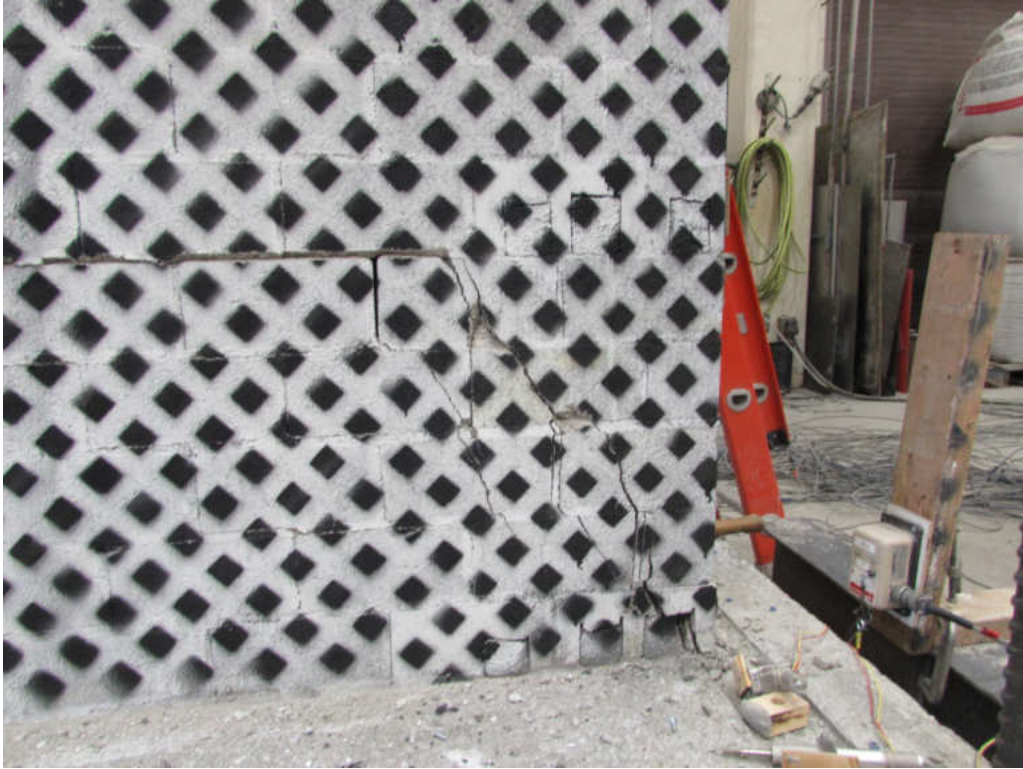
Figure 3-18: Cracking Through the Grouted Cells
