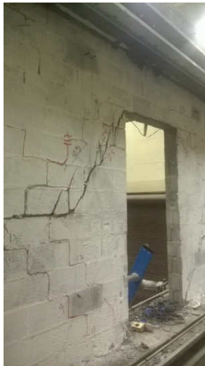
Figure 3-12: Marking Cracks During Testing
