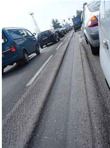
Figure 2.1. On a road between Katowice and Częstochowa in Poczesna, a large 14 cm rut is clearly visible(Wikipedia, 2019)
