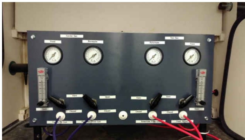
Figure 123: Front of manifold
