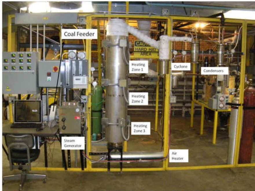
Figure 22: Constructed fluidized bed reactor system.
