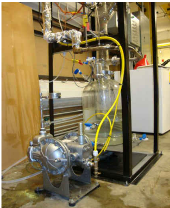
Figure 5: Diaphragm pump and scrubber 30 L tank
