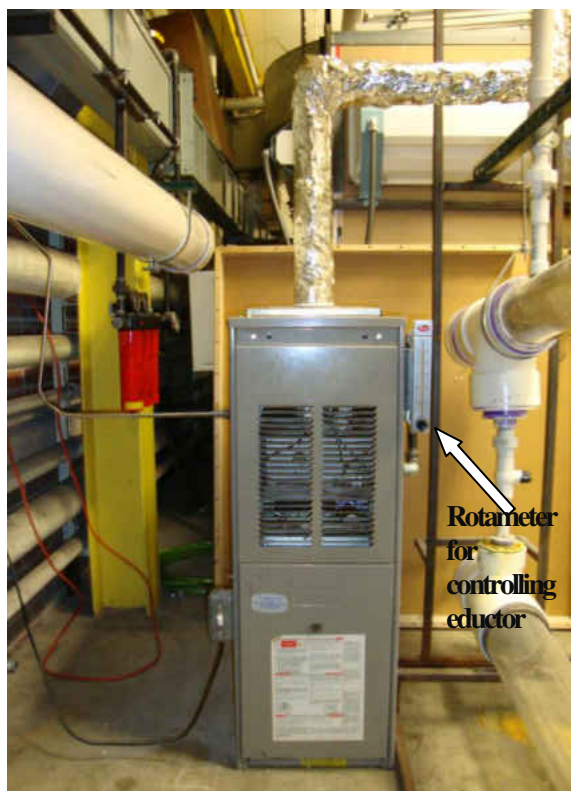
Figure 2: Modified furnace and rotameter controlling eductor
