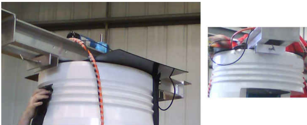
Figure 7.9: The well head to be scanned
