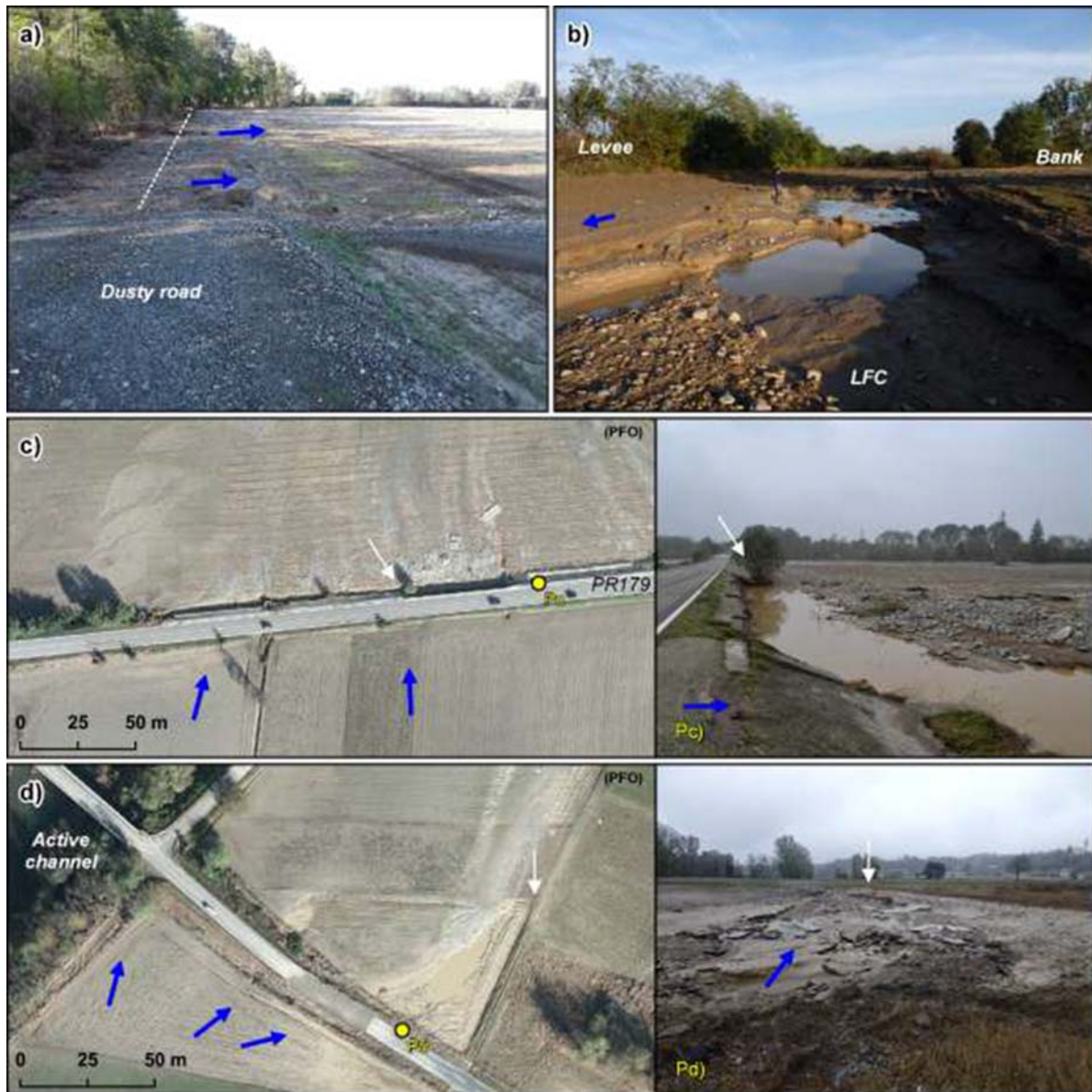
Figure 5. Effects of erosion and deposition processes over the floodplain. (a) Dusty road removed by the flood (white dotted line) and sediment lobes formed downstream. (b) Evidences (worked-soil removal and elongated scour hole formation) of intense superficial erosion that affected agricultural areas within the LFC. (c) Damage to the 179 Provincial Road embankment. (d) Damage to the road between Capriata and Bruno/Ospedale and elongated scour hole downstream of the road itself. These linear infrastructures (c, d) were overtopped and eroded. Downstream intense erosion and deposition processes occurred. It is noteworthy the draining-pipes-induced erosion downstream of the embankment (d). The white arrows (c, d) indicate the same point on the post-flood orthophotograph (PFO) (ADBDPO, 2019) and the field photograph (Pc, Pd); the yellow dot represents the location of photographs (Pc) and (Pd). The blue arrows indicate the main flood-water direction.
