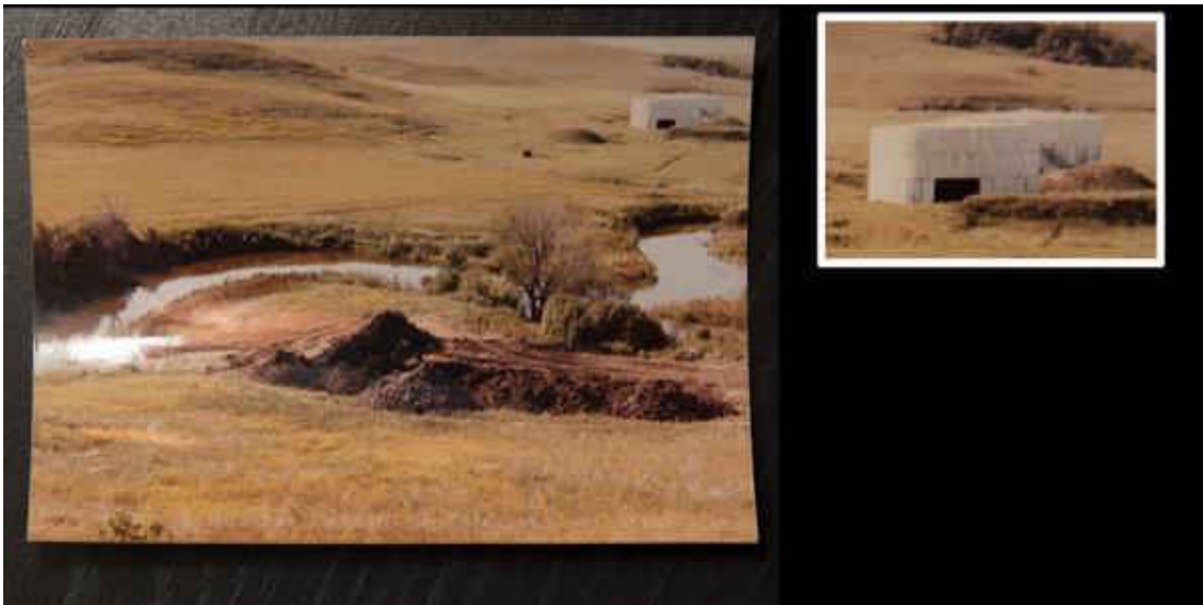
Figure 24. Participant Cody’s 1987 image a pipeline break at creek on his land. Inset image is a closer view of oil storage tank still abandoned in 2015. Cody is concerned because his cattle can enter through the opening created by a collapsed panel in one tank.
