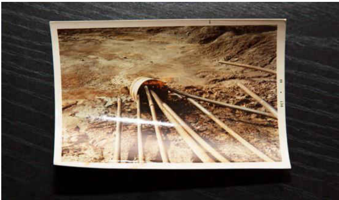
Figure 10. Flare pit. October 1969 print of an image by Cody's father that shows an early "flare pit" where pipes venting natural gas from several wells are brought together and burned off inside a barrel on the ground.
