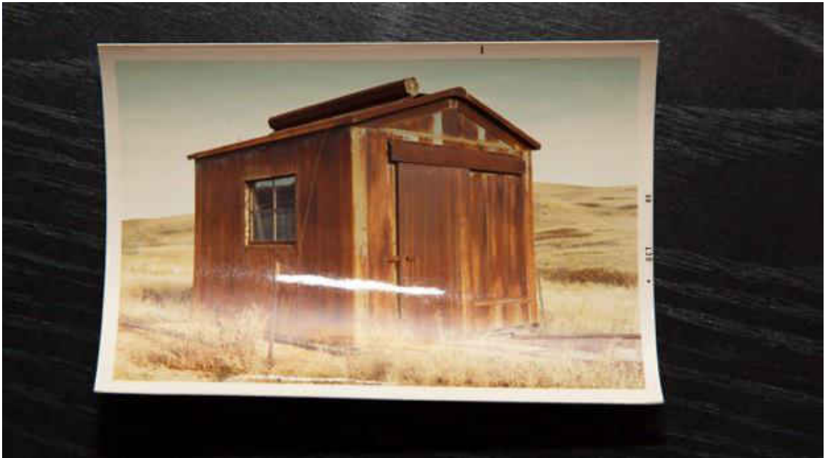
Figure 11. Metal shed oxidized by exposure to hydrogen sulfide gas. This print of an image by Cody's father dated October '69 shows a storage shed on family land severely rusted by H_2S gas.
