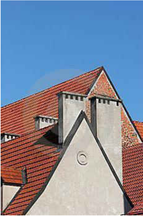
Figure 172: "Lines of Roofs"
