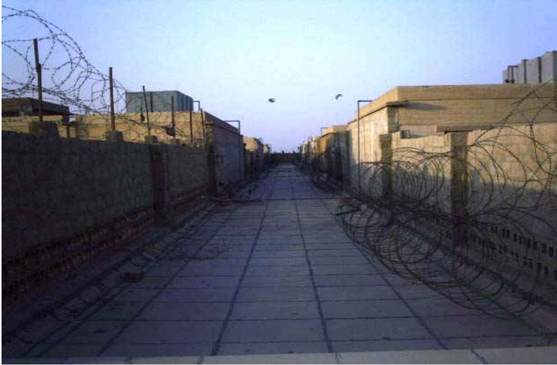
Figure 30 ~ Rooftop of Hard Site
