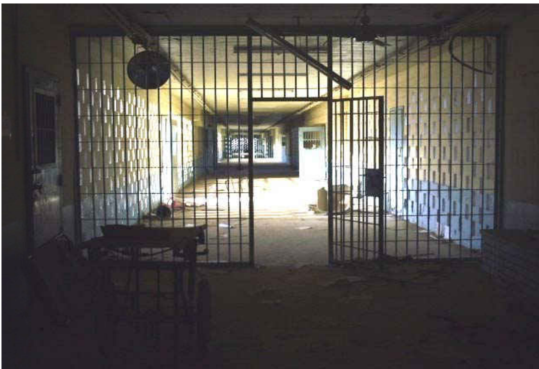
Figure 33 ~ Hallway Inside Hard Site Building
