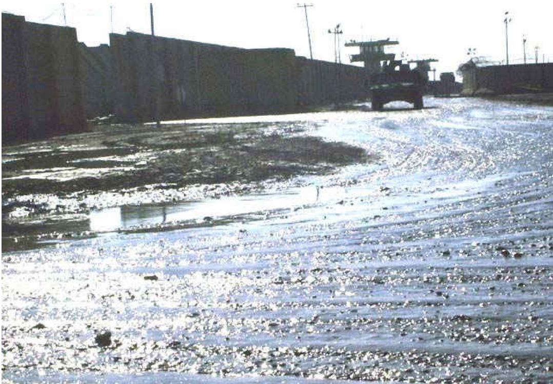
Figure 9 ~ Mud on top of the Paved Road at Abu Ghraib
