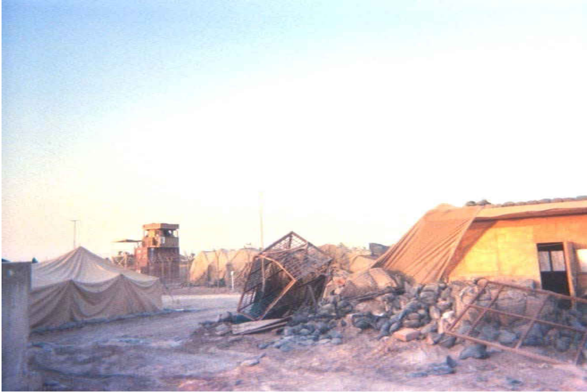
Figure 18 ~ Demolition of Compound
