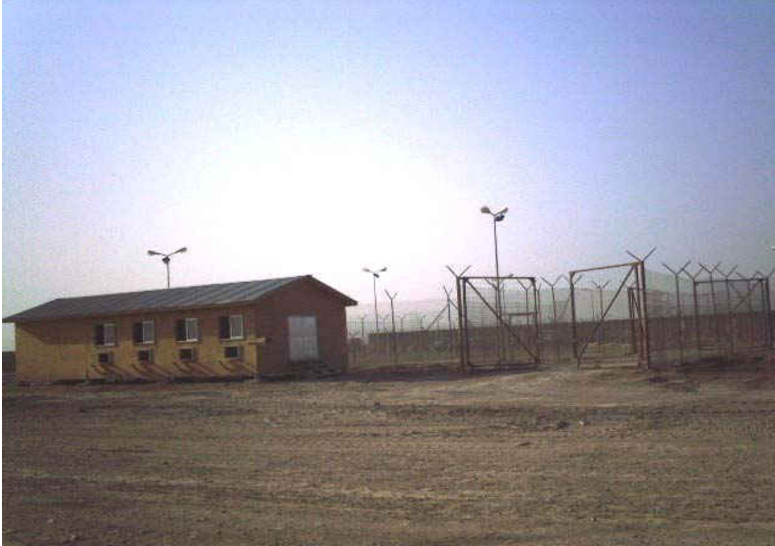
Figure 22 ~ Sergeant of the Guard (SOG) Office
