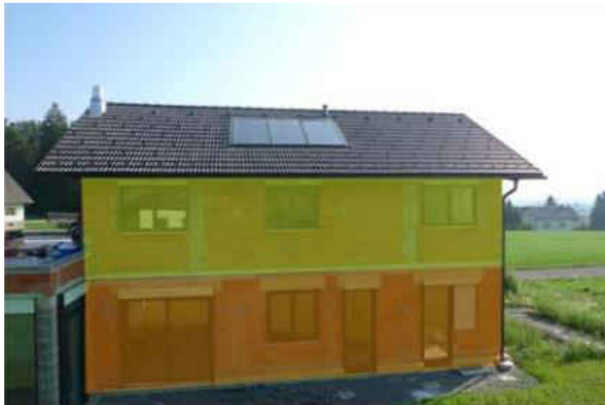
Figure 14: Construction Site Monitoring
