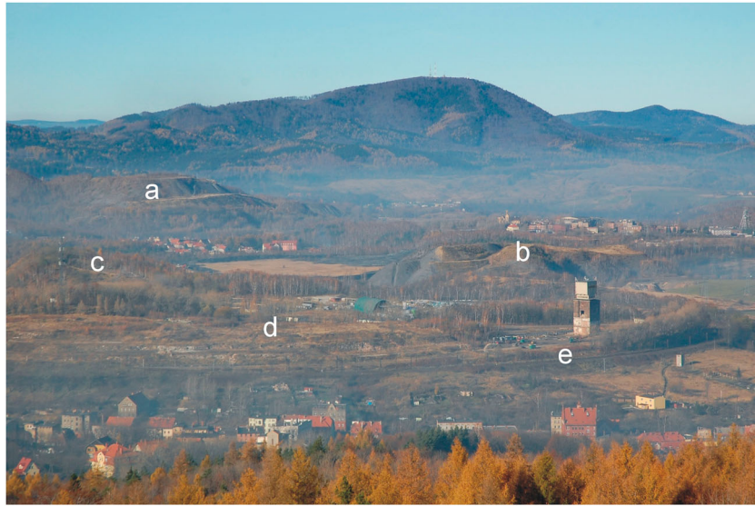
Figure 3. Contemporary view of the southern part of Wałbrzych. Notice large spoil tips (a, b, c), levelled ground left after demolition of a mines and coking plant (d) and railway embankment (e).
