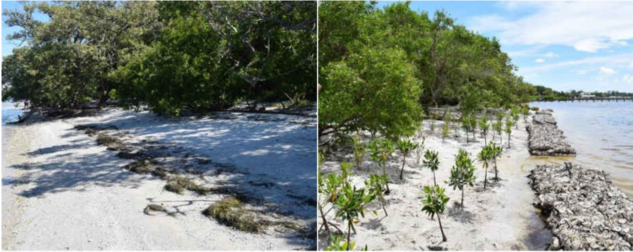
Figure 2: Example of shoreline at De Soto National Memorial before (left) and immediately after (right) living shoreline stabilization.
