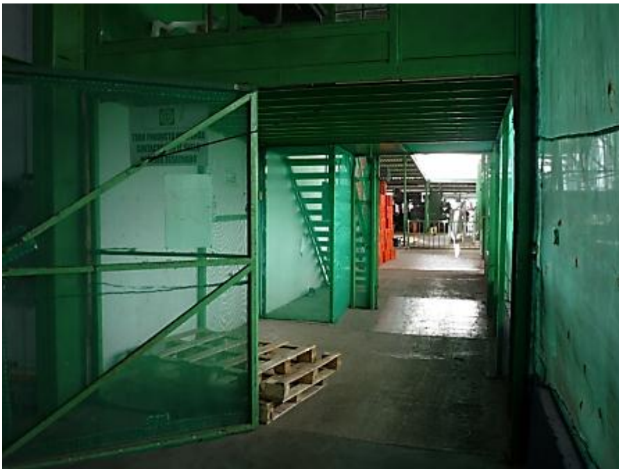
Figure 6-9 Double screen doors in a packinghouse in Escuinapa, Sinaloa, Mexico Both doors are left open in this picture taken during an off-season (Photo by author)
