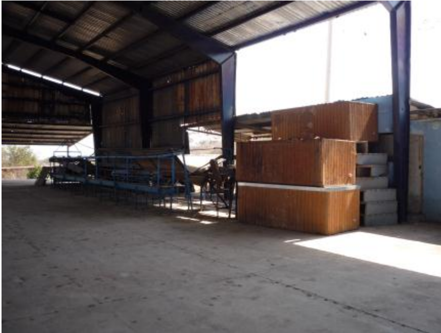
Figure 10-7 Inside of the abandoned packing facility Containers (“bathtubs”) were reminiscent of the uncompleted construction of HWT equipment. (Photo by author)
