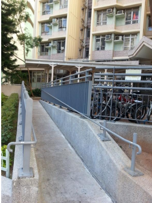
Ramps in Fu Tai estate
