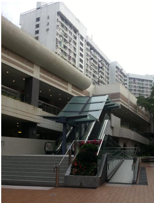
Elevators in Leung King shopping centre
