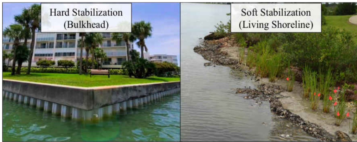
Figure 1 Image of hard stabilization versus soft stabilization.
