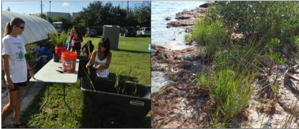
Figure 6 Volunteers potting S. alterniflora to be used for stabilization (left) and a stabilized shoreline containing planted S. alterniflora after 9 months (right).
